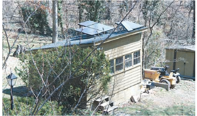
Fill ‘er up! The tractor getting topped off with solar electricity.
